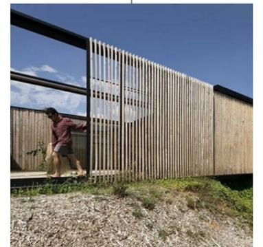
Adjustable sliding timber screens around terrace edge to protect from prevailing north-eastern winds in Summer
