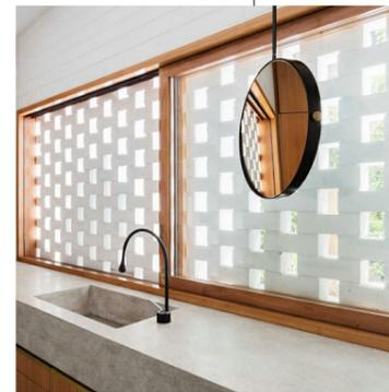
Bathroom windows with breeze block and glass screening to filter light & provide privacy
